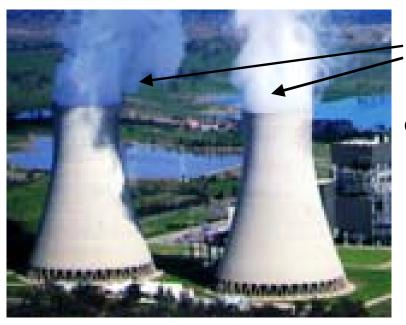
These white clouds (often falsely shown on TV as an example of "greenhouse gas pollution") consist of harmless steam coming from the powerhouse cooling towers. In these towers, the high pressure steam used to drive the turbines is condensed back to liquid water for re-use in the boilers.
